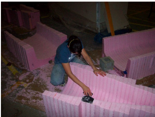
Figure 5: Sanding Formwork Sections prior to Completing Assembly
