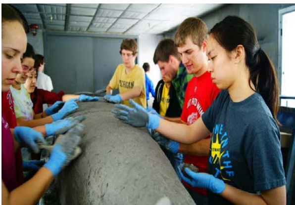
Figure 12: Hand placing of the first concrete layer on top of foam mold.
