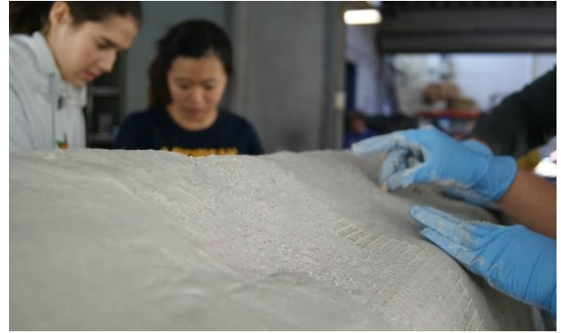
Figure 12: Placing concrete and checking hull thickness on Pour Day.
